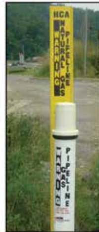
5. HCA marker and cathodic protection test station
