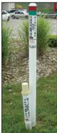
2. Linemarker and cathodic protection test station
