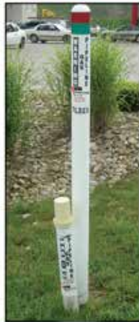
2. Linemarker and cathodic protection test station
